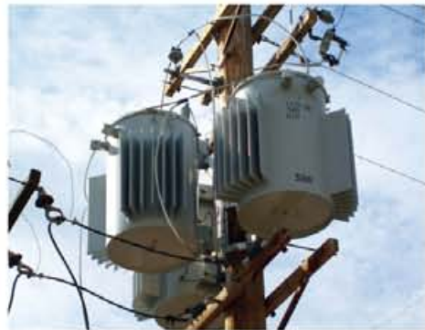
10kV~13.8kV D11型单相柱上式配电变压器 (硅钢片铁芯) Technical Data for D11 Series 10kV~13.8kV Single-Phase Pole-Mounted Distribution Transformers (Silicon Core)
