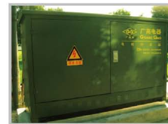
户外电缆分接箱 Outdoor cable branch box
