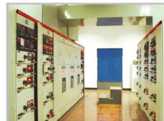
低压开关柜GCK GCK low-voltage withdrawable switchgear
