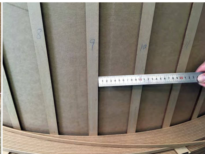
After the adhesive dispense is fixed, the span shall be corrected, and the mutual difference shall not exceed 2mm
