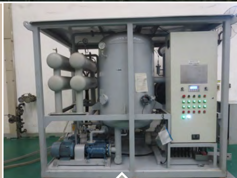
The overall air pressure leak test process is used to check the overall tightness of the transformer, and no potential leak point is spared.
